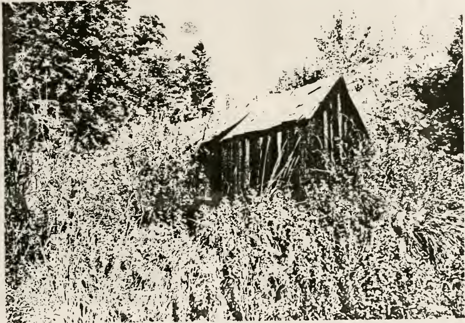
Figure 88. Revenue Mill outhouse, north view.
